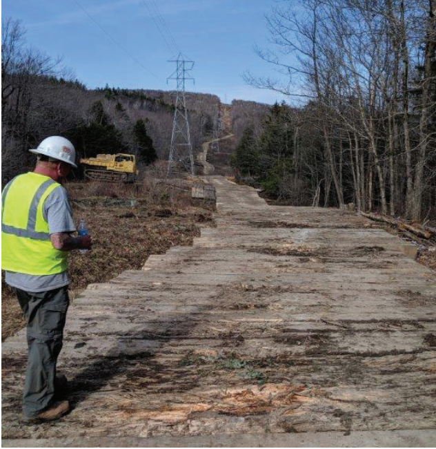
Winding temporary road
