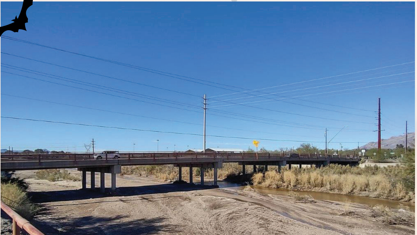
Dodge Road Bridge over the Rillito River, Tucson, Arizona.
